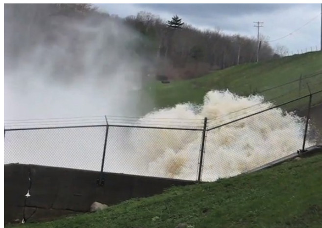
Edenville Dam spillway
